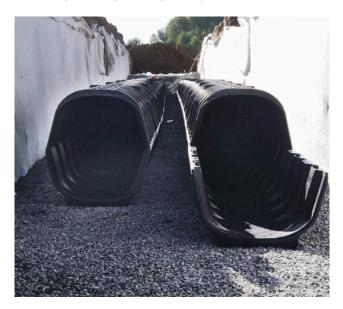
they will then form a homogenous system without cross bridges or braces within the infiltration cavity. Lay the elements and lock them into place using the connection brackets and the DRAINFIX TWIN locking device.
